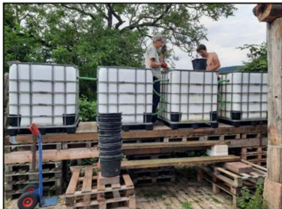
Prototyping Easy Water Filtration via the Kearns biological Filter design (2024, Niedersachsen, Germany)
