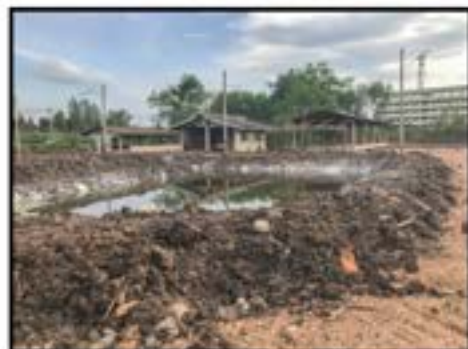
Pond Construction with Bentonite amended soil. Photo Credit: Canva
