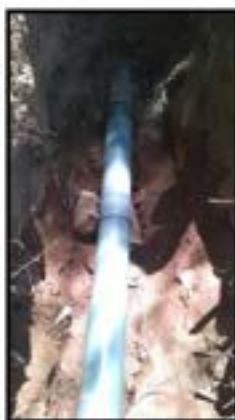
Figure 4: Pipe replaced in PVC PN16
