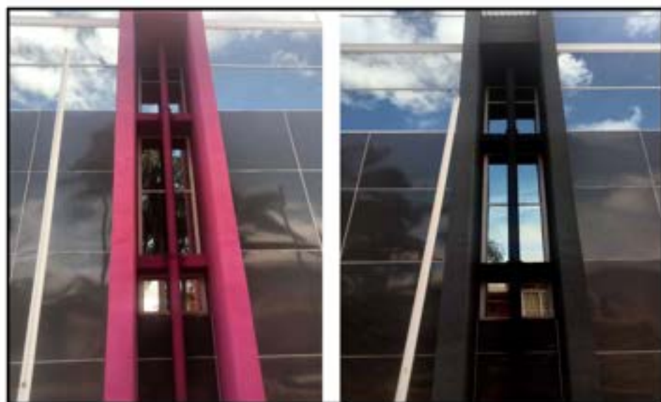
Rainwater drain pipes
