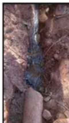
Figure 3: Fibre pipe cut 5m upstream of the sump
