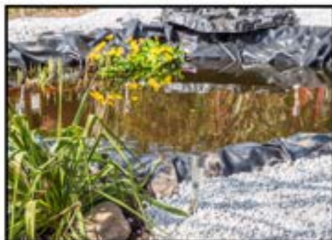
Pond Construction with synthetic Liner. Photo Credit: Canva
