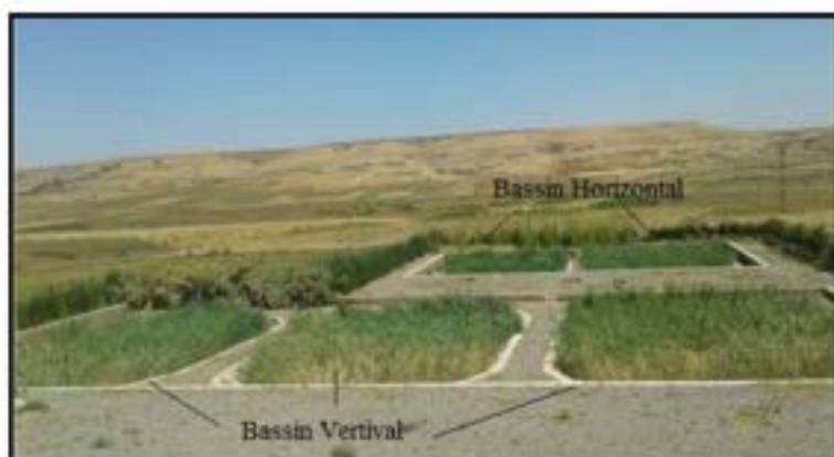
Figure 2. The two-stage CW configuration comprises three VSSF-CWs in parallel in the first stage and two HSSF-CWs in the second stage. Photo Credit: El Fanssi et al., 2019, http://www.geoecotrop.be/
