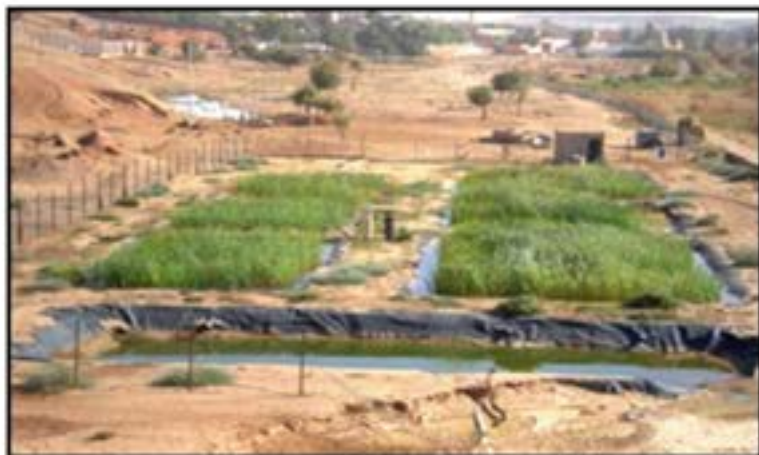
Figure 6. A wide-angle view of the hybrid system in the Brézina CW configured in parallel. Photo Credit: Bouchama, 2022, https://doi.org/10.1007/978-3-031-03600-2_2
