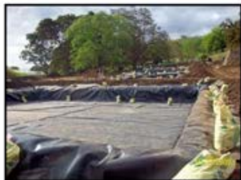
Figure 16. The Q-Sem Seed Farms CW with black linings laid out to prevent wastewater leakage into surrounding ground areas. Photo Credit: GreenWater, https://www.green-water.org/clients/
