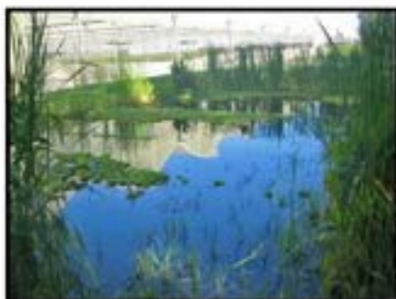
Figure 17. The Tambuzi Flower Farm CW with papyrus and water hyacinth reed beds. Photo Credit: GreenWater, https://www.green-water.org/clients/
