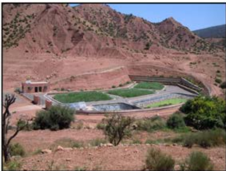
Figures 4. An aerial view of the Asselda CW. Photo Credit: Engeli, 2016, https://www.eawag.ch/en/info/portal/news/news-archive/archive-detail/bouziane-outiti-wins-energy-globe-award-for-wastewater-treatment-project/
