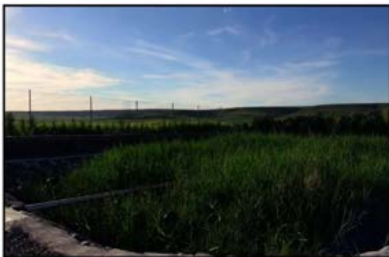
Figure 3. One of three VSSF-CWs constituting the first stage of the Tidili Mesfioua HCW. Screenshot Credit: YouTube, https://www.youtube.com/watch?v=a3xVM7VdoWk
