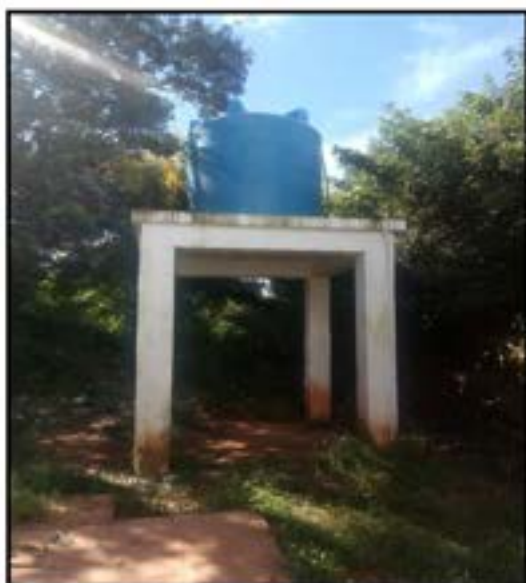
FIGURE 8 : An tank near the swimming pool with the volumes : 5000 liters
