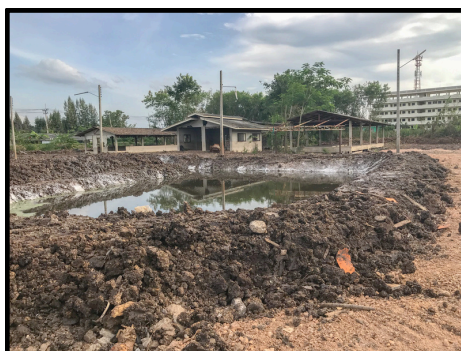
Pond Construction with Bentonite amended soil. Photo Credit: Canva
