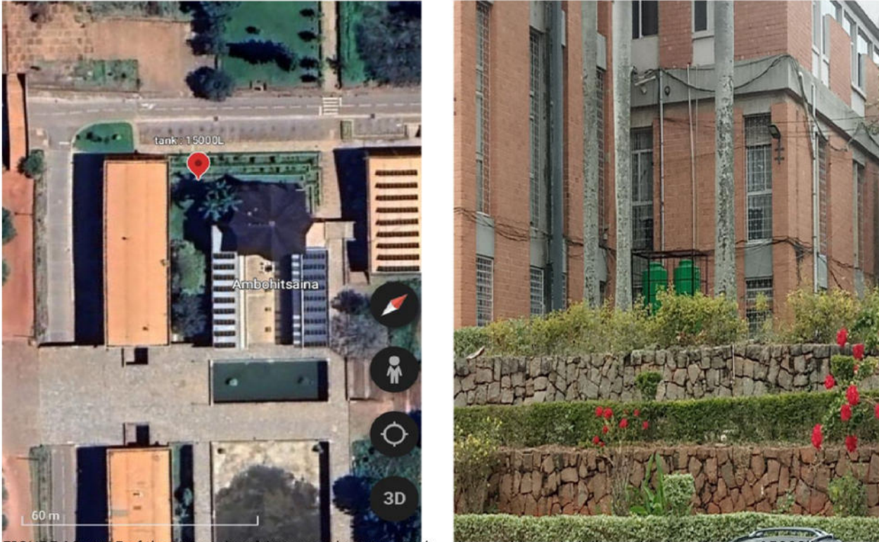
FIGURE 10: MAP of the University of Antananarivo : An tank in « the presidency building »with the volumes : 15000liters The storage at the presidency has a capacity of 15000liters and supplies water to several faculty.
