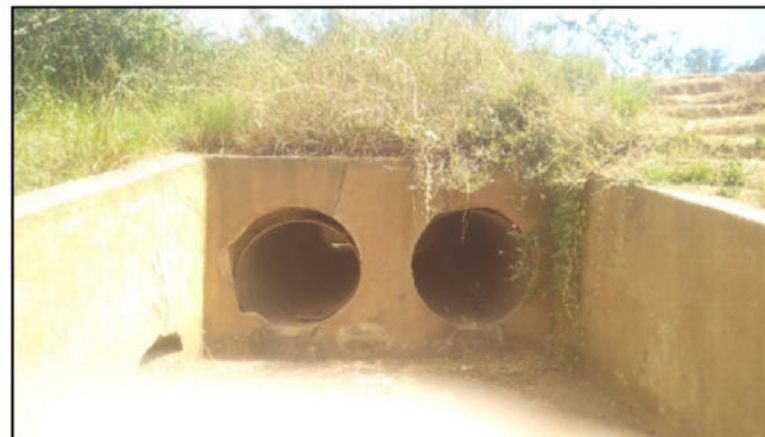
Figure 4: Stormwater Runoff being routed to the Rice Fields (Zone 1) Photo Credit: FINARCH
