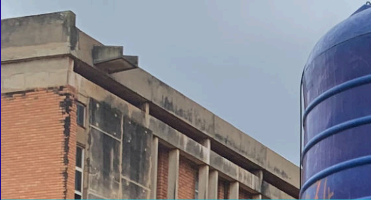
Figure A: Sciences Building
